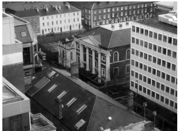
Bird's eye view: Historic May Street Church as seen from the Belfast Eye - a good opportunity to check over the roof. Photo: Robin Morton.
